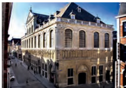
De Hallen at the Naamsestraat can be considered as the headquarter of KU Leuven. It was originally used by weavers for selling cloth. Shortly after the establishment of the university (in 1425), the city put part of the building at the disposal of the colleges as a classroom. The building currently serves as the university's administration centre. It is still the central place of student enrolment, and one of its halls is still regularly used for public PhD defences.
